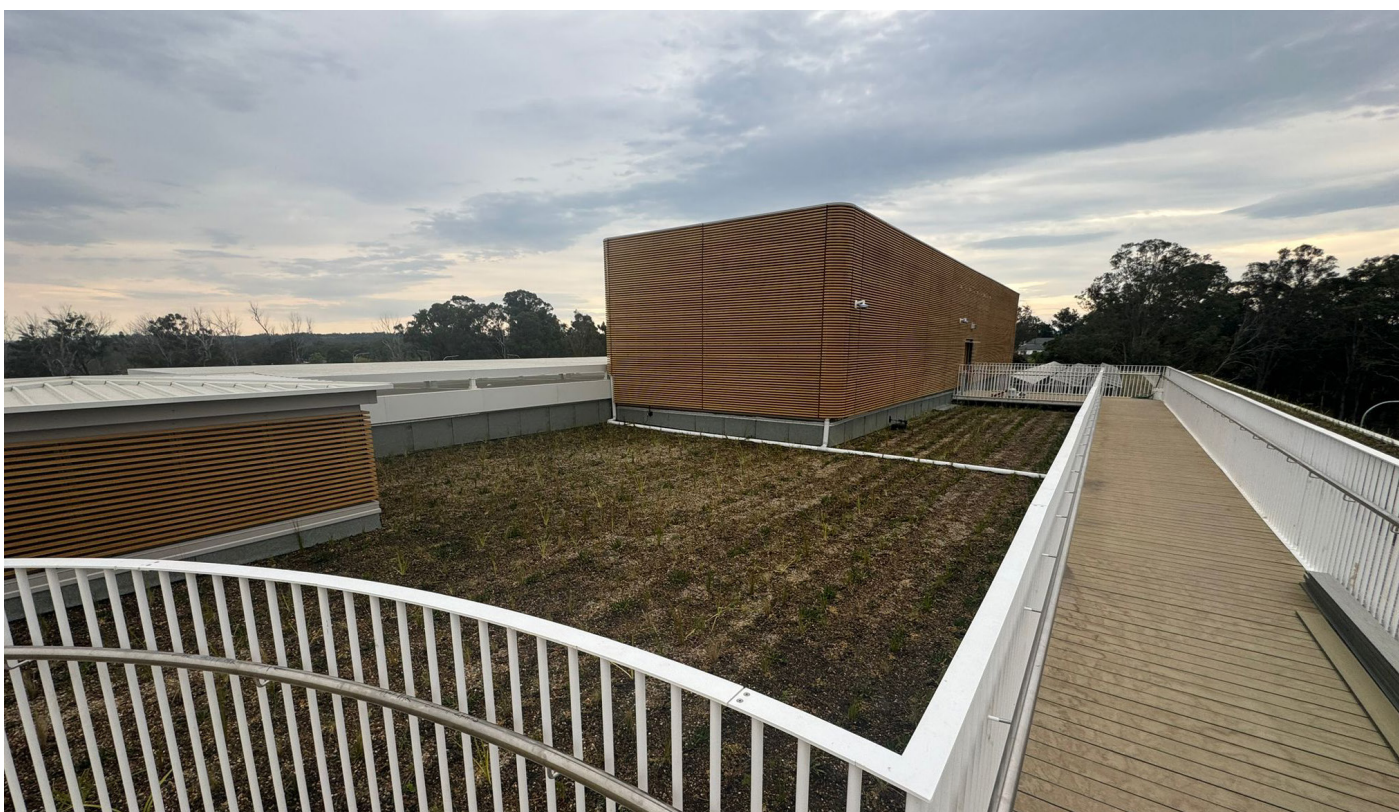
FINISHED GREEN ROOF
