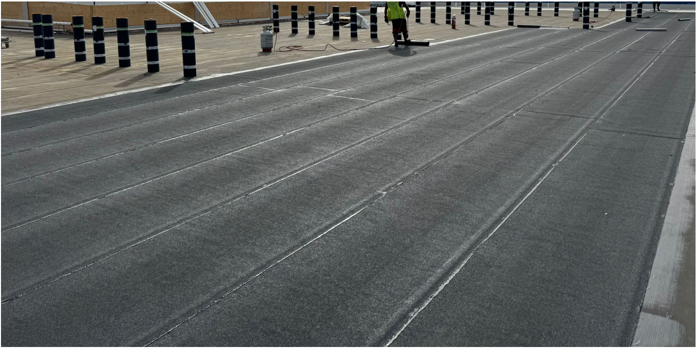
UNDER METAL ROOF CAP SHEET
