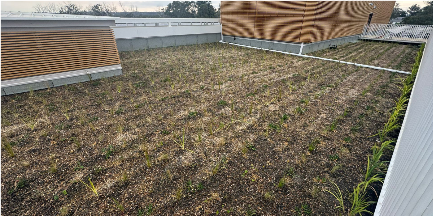
FINISHED GREEN ROOF
