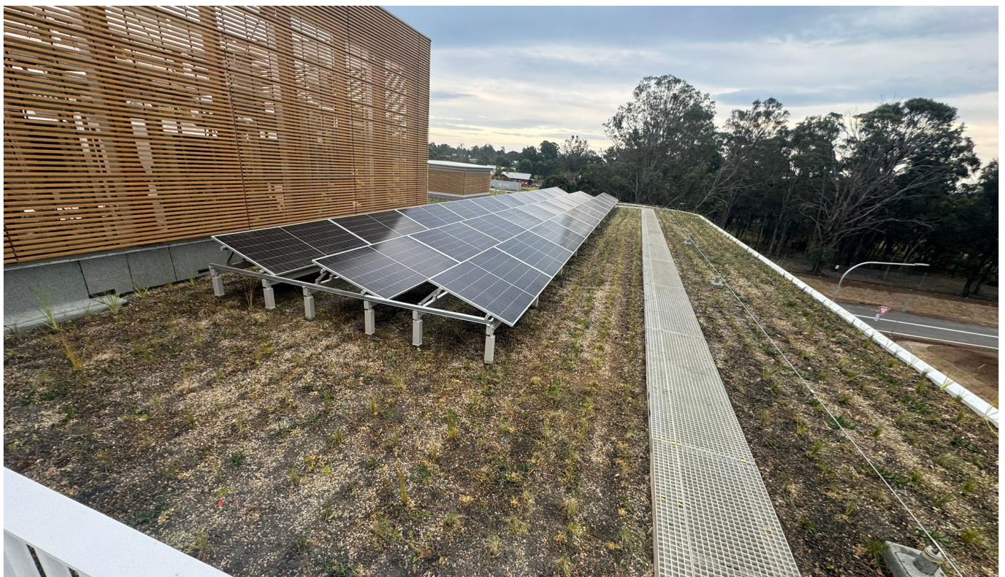
FINISHED GREEN ROOF
