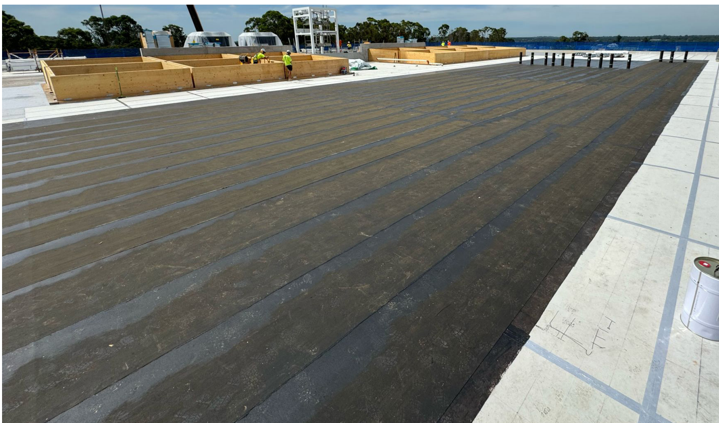
UNDER METAL ROOF BASE SHEET
