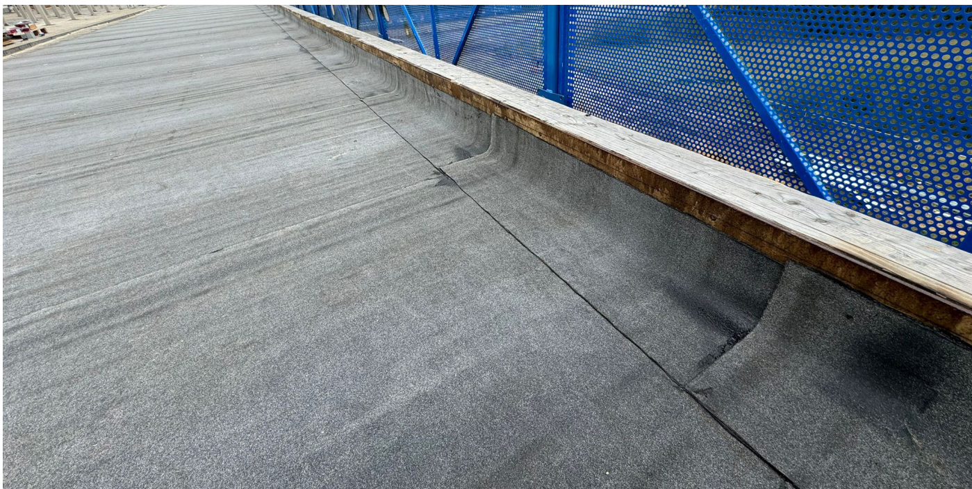
PERIMETER METAL ROOF BASE SHEET
