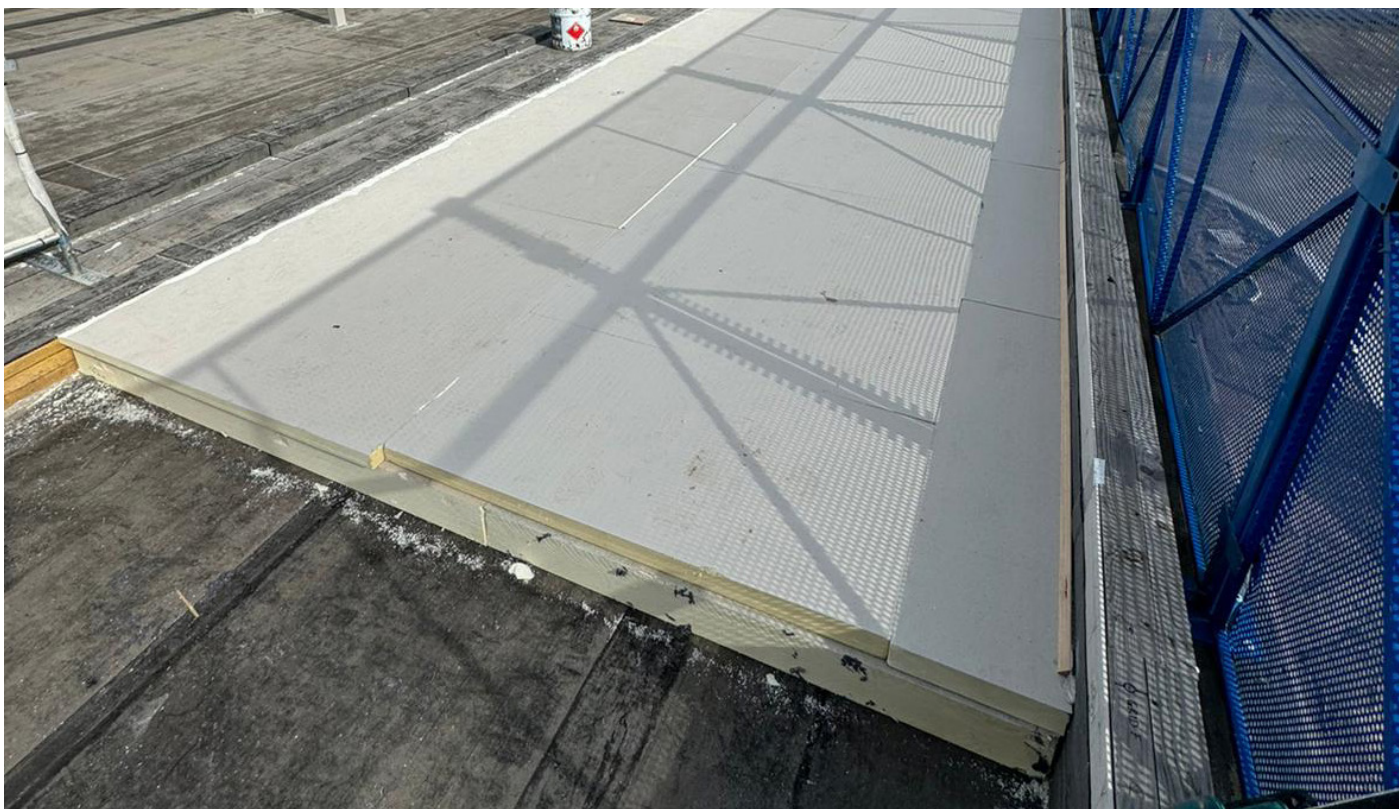
PERIMETER METAL ROOF INSULATION
